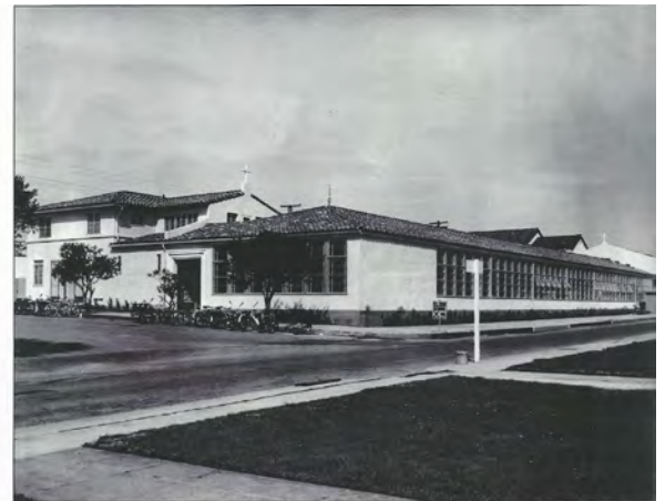
ST. PATRICK'S SCHOOL COMPLEX, 1949. Expansion of the school, a convent for the teaching nuns, and additional playground space remained a vision for the parish. The new complex of school buildings, a parish hall, and convent opened in the fall of 1949, with seven nuns teaching 254 students in eight grades. This view is along Ray Street to the right at Capps Street. (Courtesy of St. Patrick's Church.)
